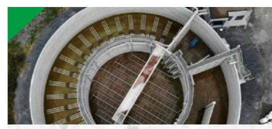
A new-generation wastewater treatment plant, HYBAS™, is currently under construction at COSUCRA. This fixed biofilm treatment plant aims to offer better purification performance for our industrial water than our current activated sludge basins. Commissioning is scheduled prior to end 2024.
